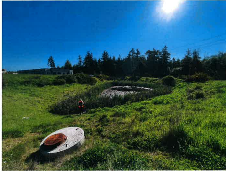
Photo 13. Stormwater retention pond facing northeast
