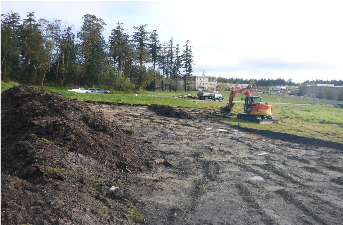
Figure 8. Logging residue spoils on the left. Gray gravelly sands exposed on the right. Operator starting 3rd Transect at the northeast corner, south of the berm. View to the northeast.
