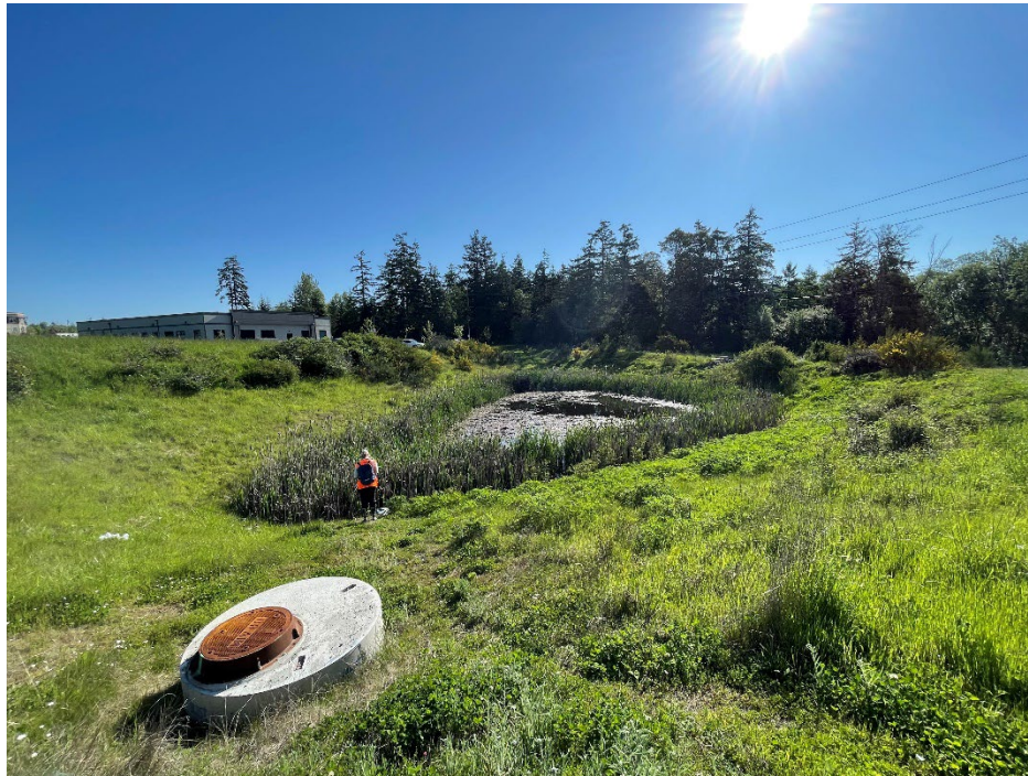
Photo 13. Stormwater retention pond facing northeast
