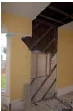
Original plank frame wall and diagonal lath and bracing. 2011
