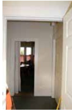
First floor hallway. 2011
