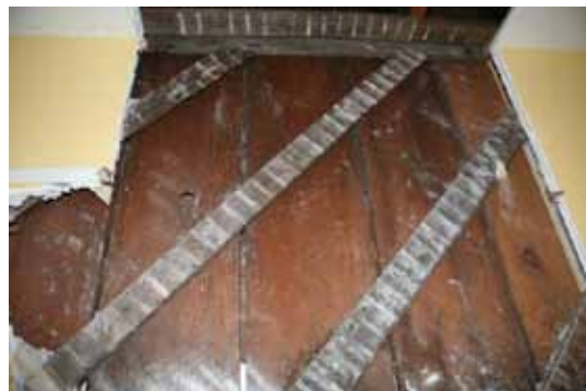
Detail of original wall framing. 2011
