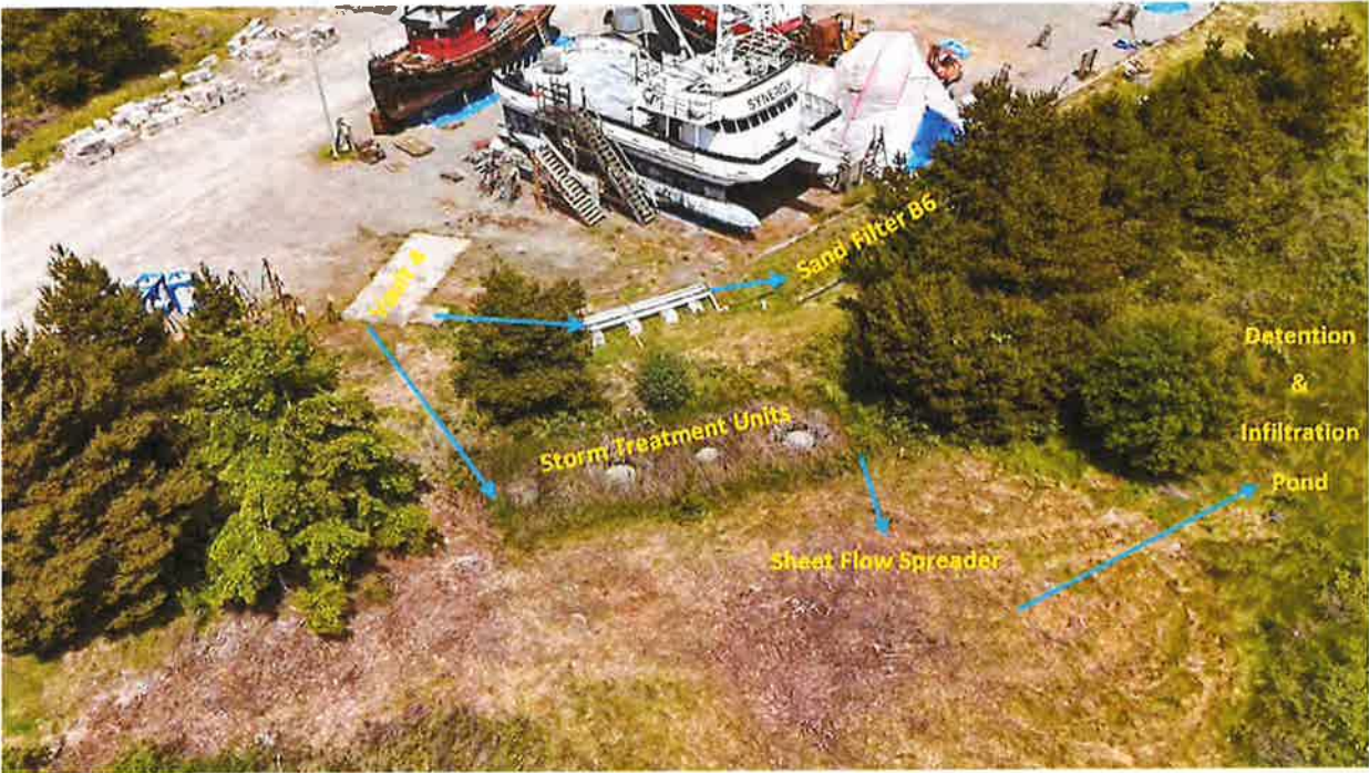
Photo 3. The existing Port Stormwater Facility (center) is located at the northern margin of the study area, adjacent to the Boatyard. Stormwater from the facility discharges to the depression (far right) for detention and infiltration, as evidenced by the green vegetation. The wetland buffer ends at the southern edge of development as the Boatyard and Port Stormwater Facility effectively preclude the function and value typically derived from wetland buffers.
