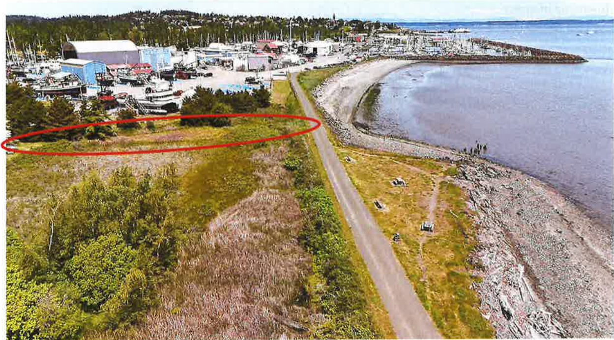
Photo 5. Study area facing north. The flow spreader embankment (circled in red) stretches from 8th Street to the Larry Scott Memorial Trail, separates Wetland A from the Boatyard. The Study Area is confined by 8th Street (left) and the Larry Scott Trail (right).
