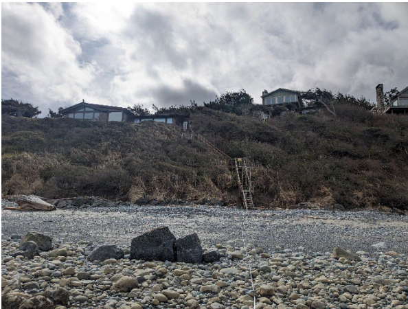
Photograph 1. View of the bulkhead and residences from the shoreline, view to the southwest.
