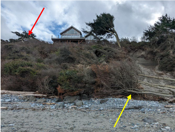
Photograph 8. Yellow line points to end of bulkhead on west-adjacent property at the start of the landslide and red arrow points to residence on West Lot, view to the south.
