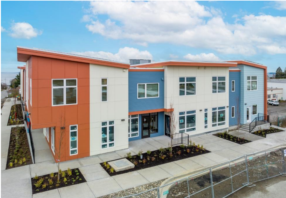
7 th Haven Low-Income Housing project at Hendricks and Seventh Street in Port Townsend.
